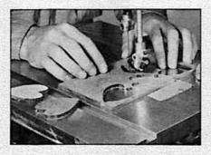
Jig Setup For Doweled Miter Joints
